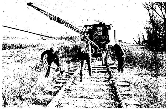
WORKMEN remove the last few miles of rail between Norfolk and Wayne, ending the role of the railroad in development of this part of the state.
